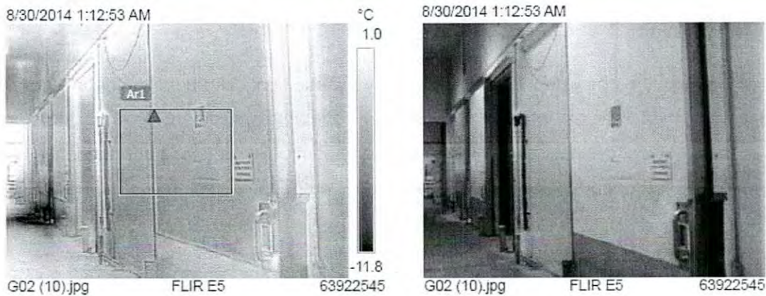
Fig. 10. Infrared assessment at the company
